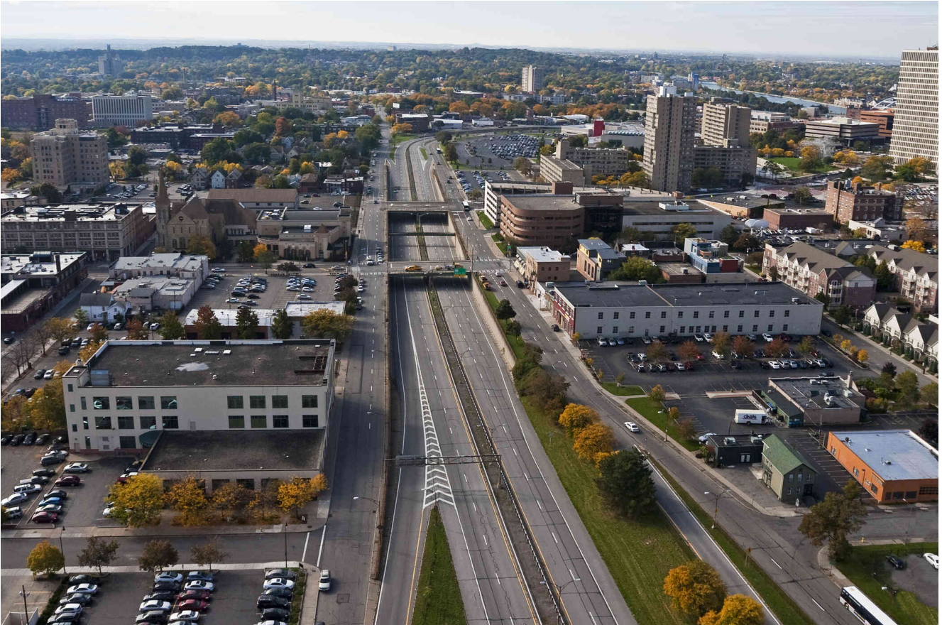
The eastern section of Rochester's Inner Loop highway, before it was removed. City of Rochester
